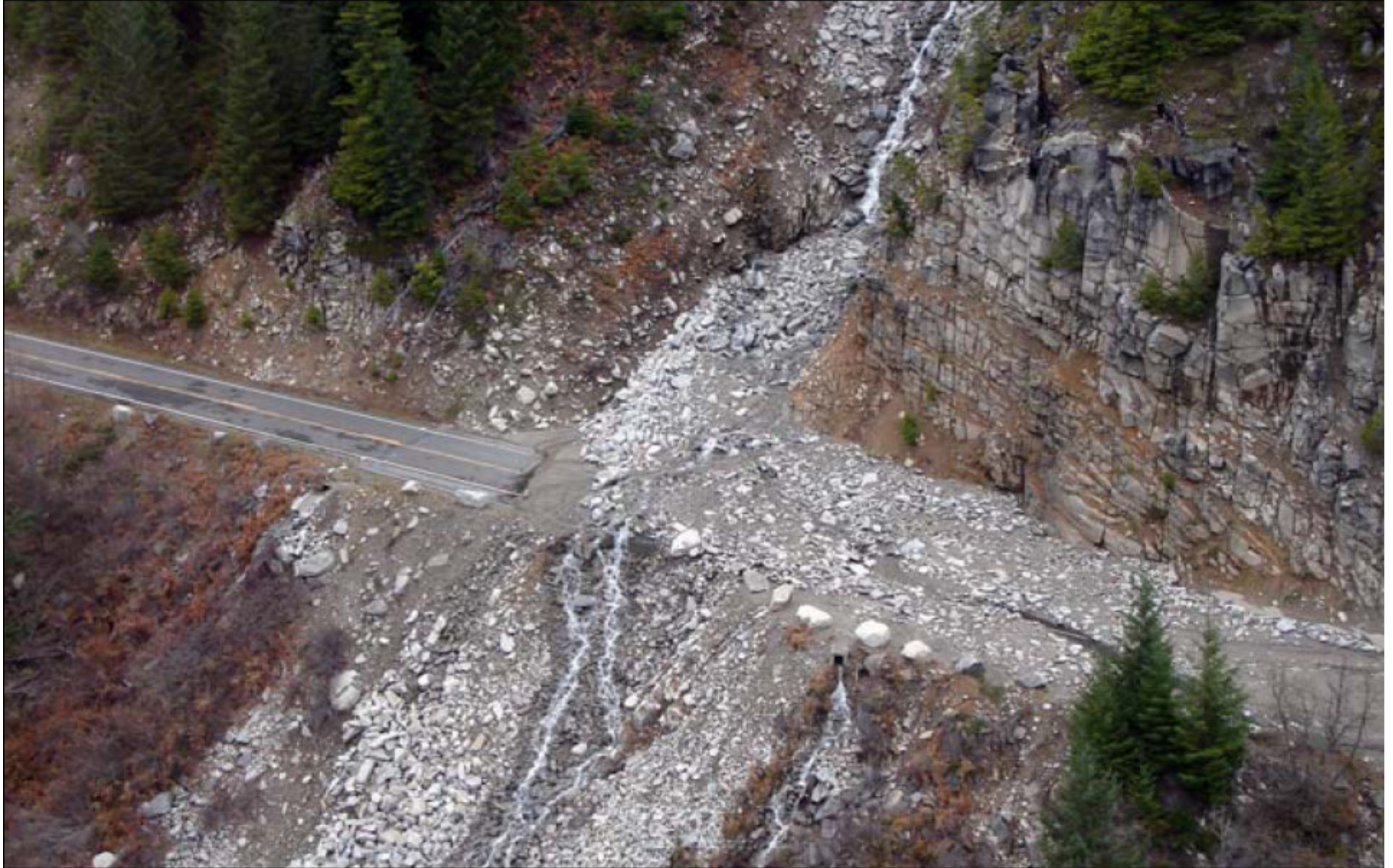
Landslide below Stevens Ridge in Stevens Canyon
